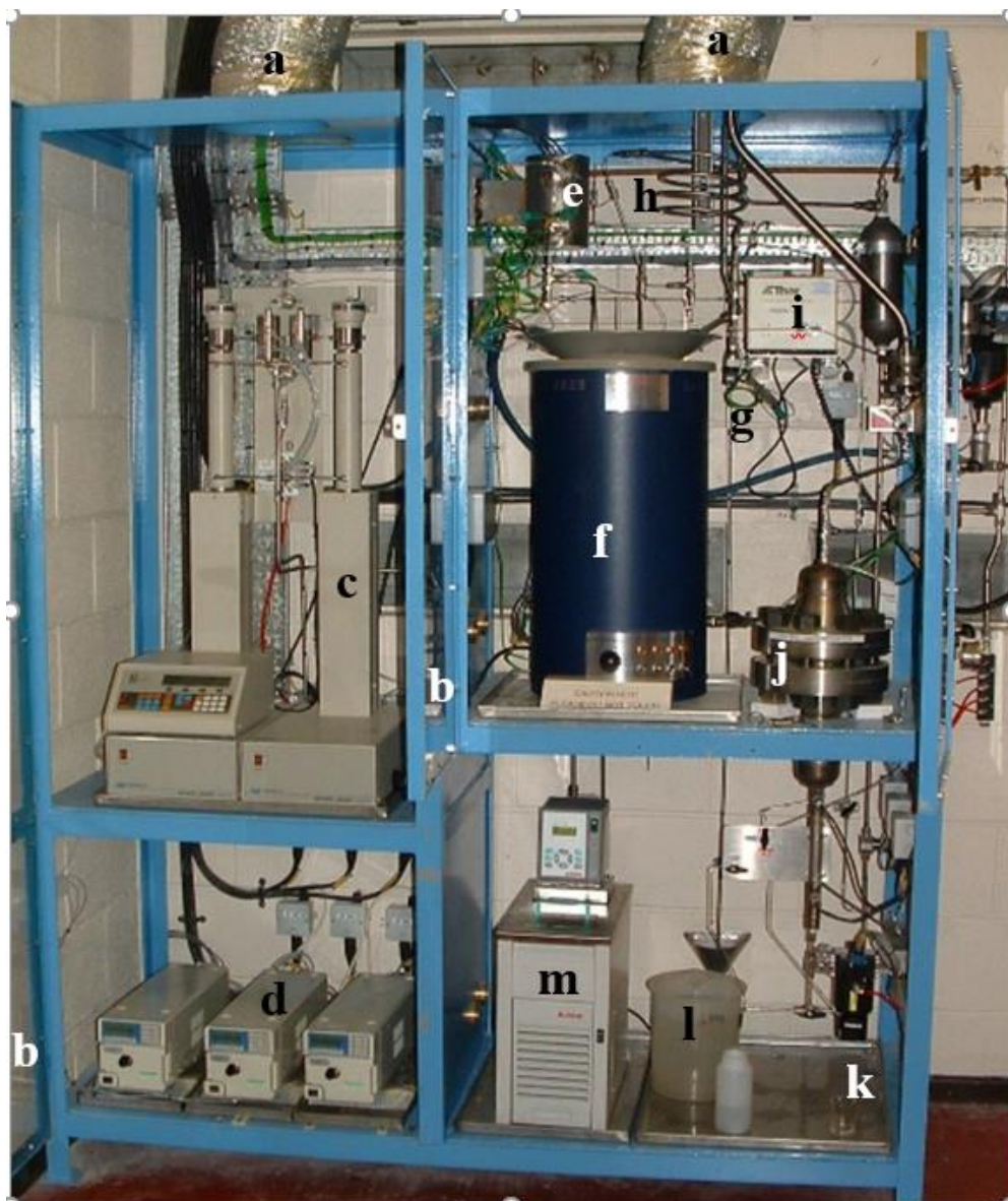
Figure 2-7. The K5 kinetics rig as originally installed. The secondary containment cabinet is constructed of (blue painted) steel with polycarbonate sheeting and has extraction visible at the top (a). Hinged doors to enable cabinet closure can be seen to the left and centre (b). The feed vessels are mounted on a rack to the left of the camera position and are out of shot. The ISCO twin syringe pump for pX can be seen in the top left cabinet (c) and three Jasco HPLC pumps (d), for catalyst solution, peroxide solution and quench solution, are in the bottom left cabinet. The reactor cabinet is top right and a description of its contents follows. The pre-heater coil (e) is contained in the metal enclosing casing in the top left. The sand bath (f) is the large blue container at bottom left and the reactor is inside this. The quench point (g) is to the right and slightly above the sand bath and the cooler is the coil (h) above that. The back-pressure regulator (i) is inside the grey housing labelled ‘Thar’. The gas/liquid separator (j) is the flanged vessel at bottom right and extends down into the sampling area in the lower right cabinet. The sampling area is not enclosed (as it is at low pressure) and it is banded (k). Plastic collection containers (l) are visible. There is a Julabo temperature controlled bath (m) in the left of the sampling area that can pump cold fluid around the sand bath cooling coil. The Rosemount gas analysis unit is mounted to the right of the camera position and is out of shot.
