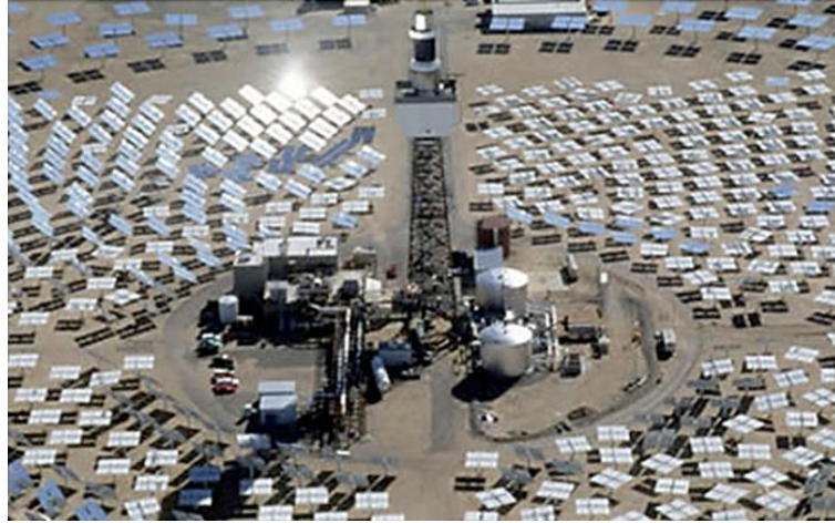
Figure 2.9: Ivanpah solar tower power plant in the US [33]
