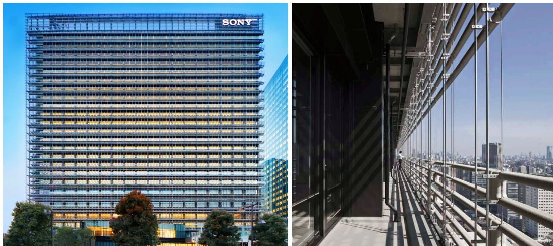
Figure 2.27 Bioskin NE façade. Sony Osaki Building, Japan (Nikken, 2011, p. 1)
