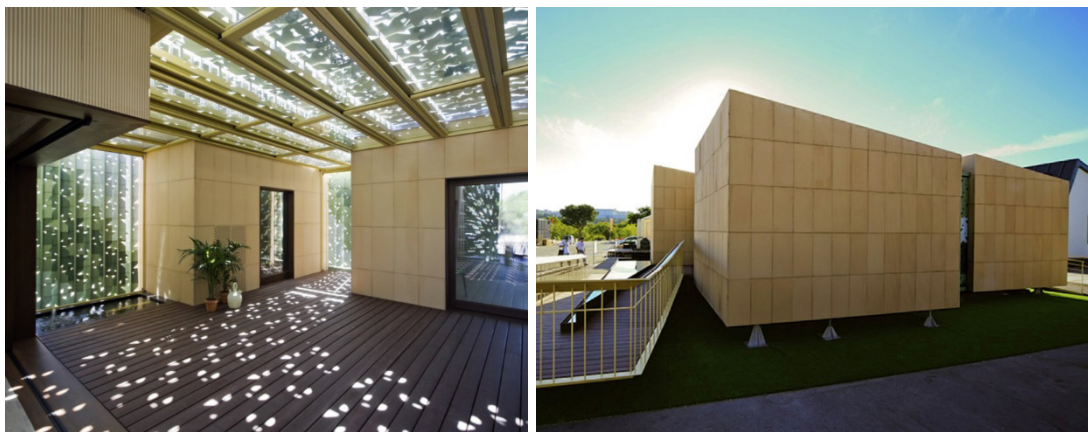
Figure 2.24 Interior and exterior view of Patio 2.12, Madrid, September 2012 (Terrados and Moreno, 2014, pp. 71, 78)
