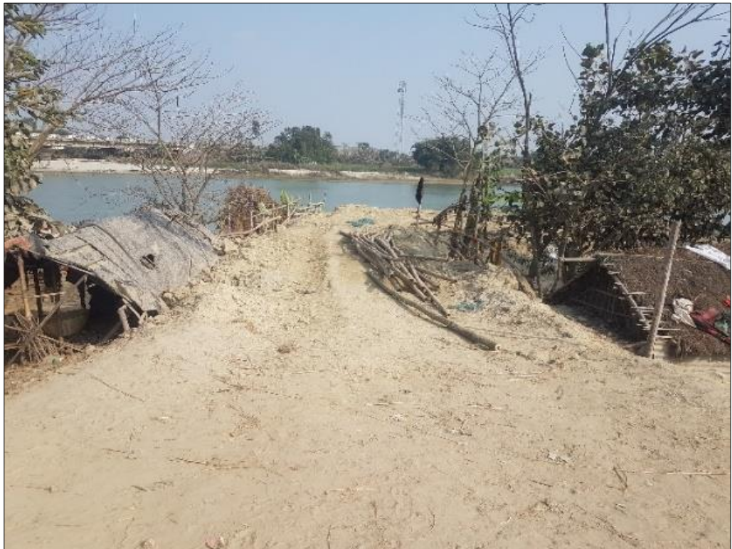
Figure 5-19 Zamindars forcefully put mud on the west embankment houses The permanent relocation of people from within embankments and waterlogged areas established that the west embankment
