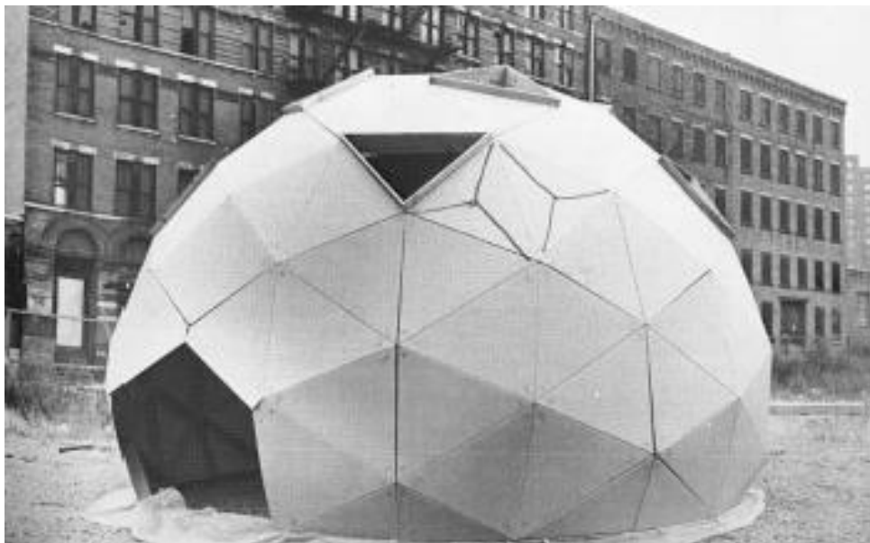
Figure 4. Geodesic Dome with Cardboard Pieces Source: Mottel, Charas: The Improbable , 35.
