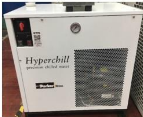
(c) Water cooled chiller
