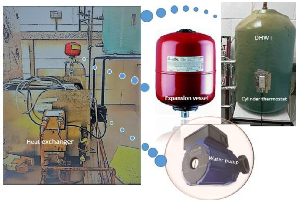
Figure 7.4. Main components of the water heating loop
