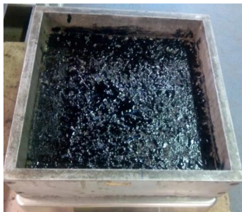
Figure 40 Tack coat application
