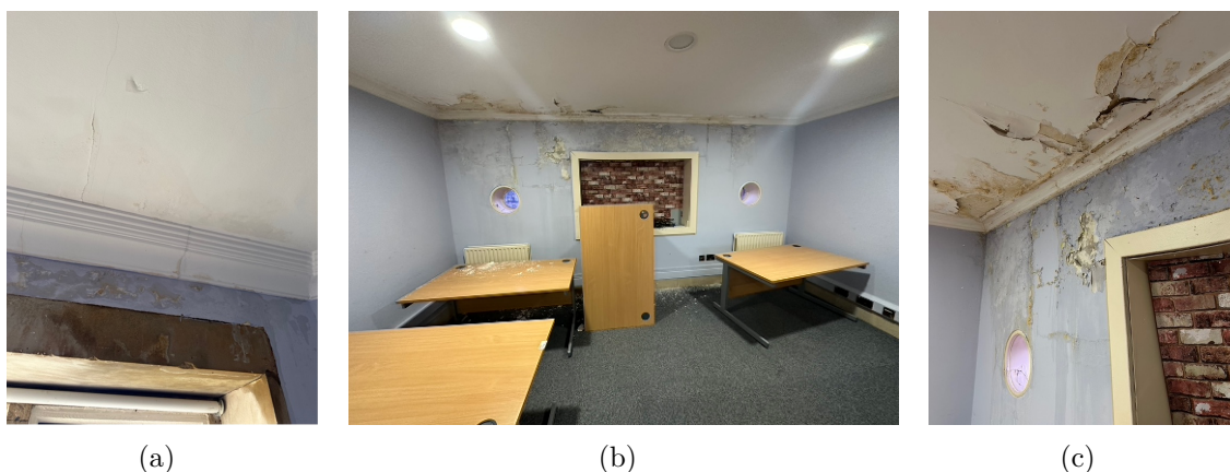
Figure A.4: Images from the internal building survey of Lenton Lodge Gatehouse. Here, the rooms behind the (a) north turret, (b) central traceried panels (the other side of the circular windows) and (c) bronze plaque (behind the brick wallpaper) are shown, with visible signs of water ingress, material decay and damage identifiable.
