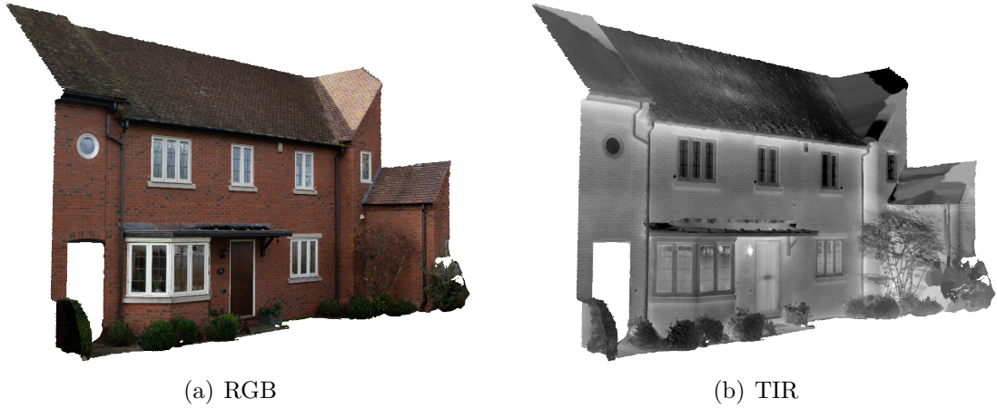
Figure 5.13: (a) RGB and (b) TIR textured 3D polygonal models for Dunrobin House.
