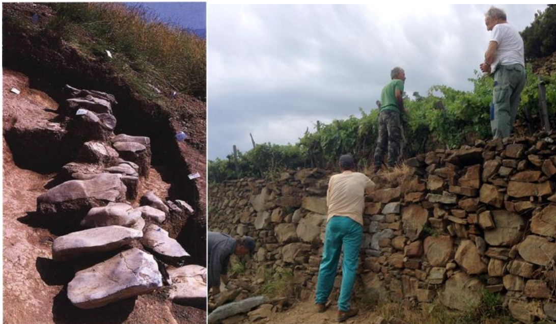
Figure 6.11 FBA terracing at Monte Borgo (GE1) (left) and modern construction of terraces in Liguria (right) (after Maggi, 1998, 126, fig. 2; Parco Nazionale delle Cinque Terre, 2021)
