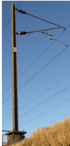
Figure 2-7 Universal Column Structure
