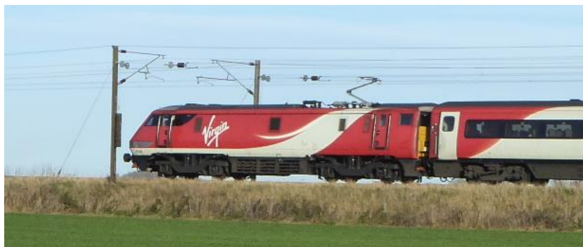
Figure 2-1 25kV AC Overhead Electrification on the East Coast Main Line South of Darlington
