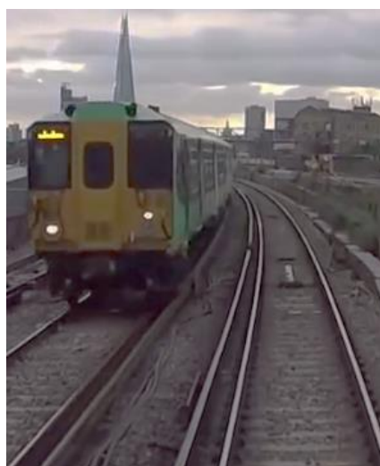
Figure 2-2 Conductor Rail Electrification on the Brighton Main Line near London Bridge (FourFoot, 2016)
