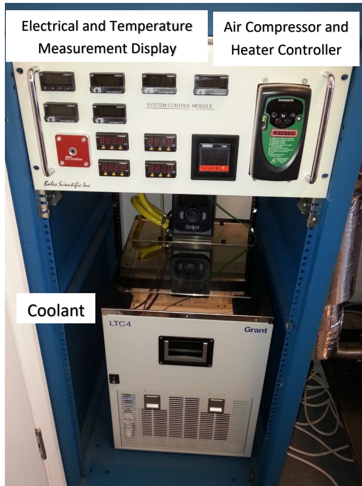
Figure 7-18 Coolant and first data acquisition unit.
