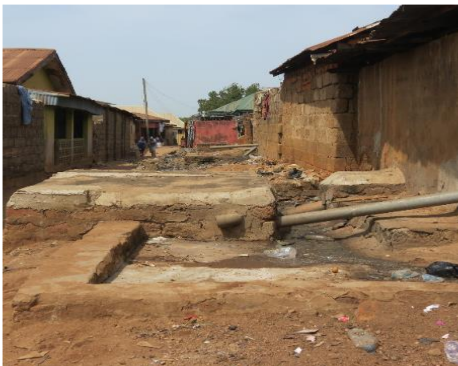
Plate 4.11 A poorly constructed toilet in Wadata Source: Fieldwork 2016
