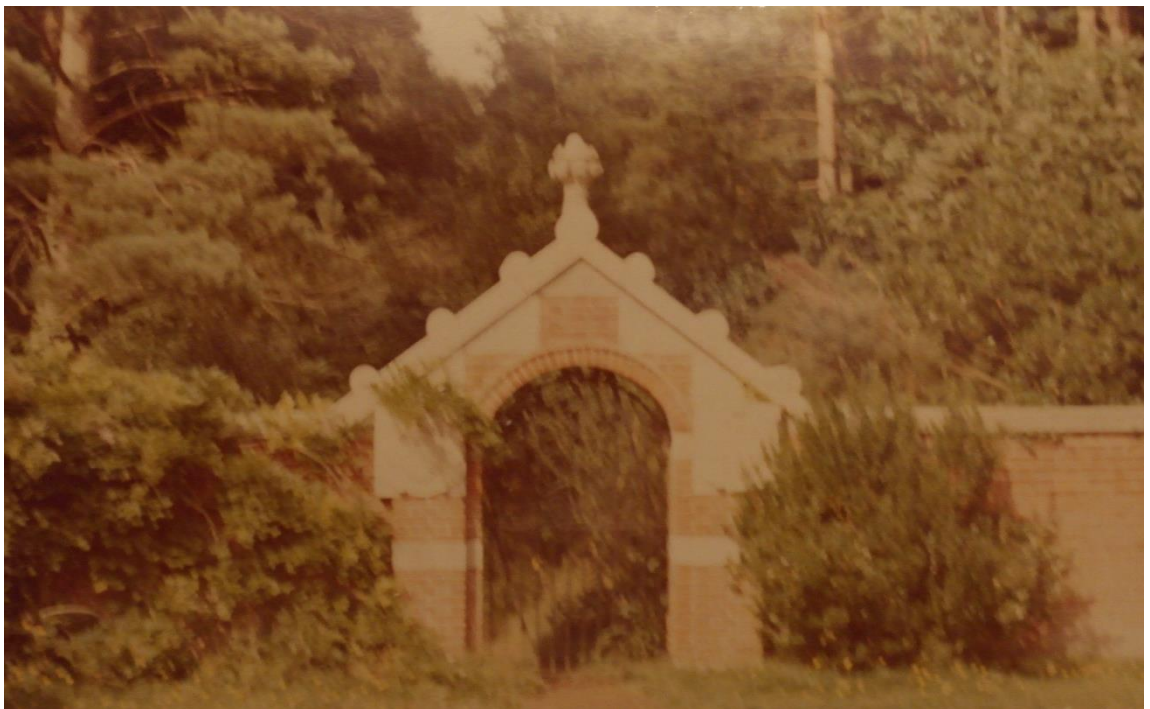
Figure 35: Arch Gateway in courtyard at Avon Tyrrell
