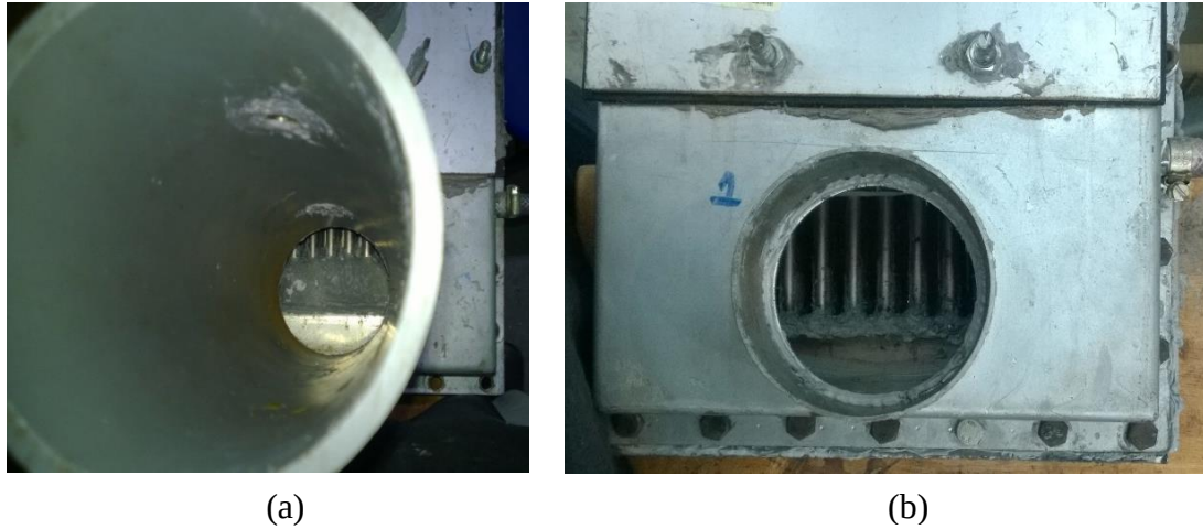
Figure A4: Appearance of the interface between the HHX and the TBV (a) before and (b) after the rectification work.
