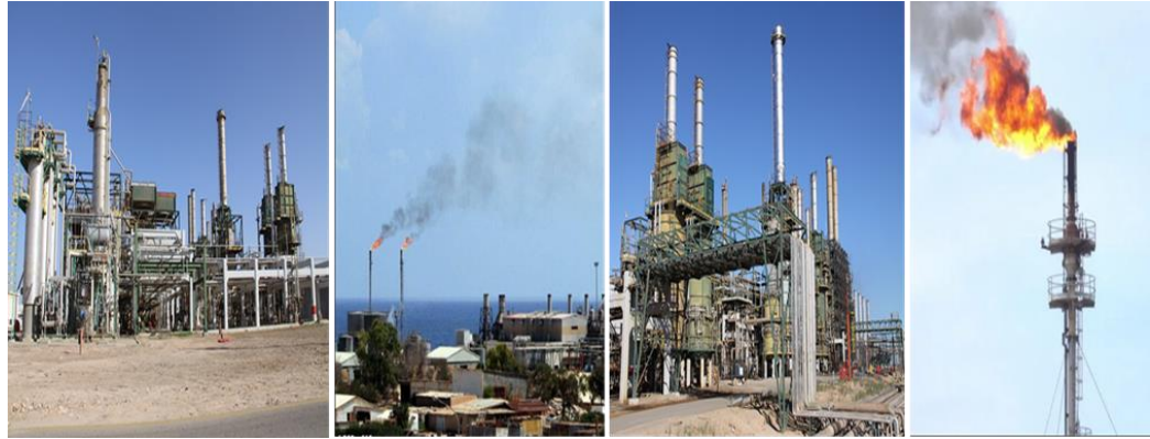
Figure 6. 2 Photos of Az Zawiyah Oil refinery.
