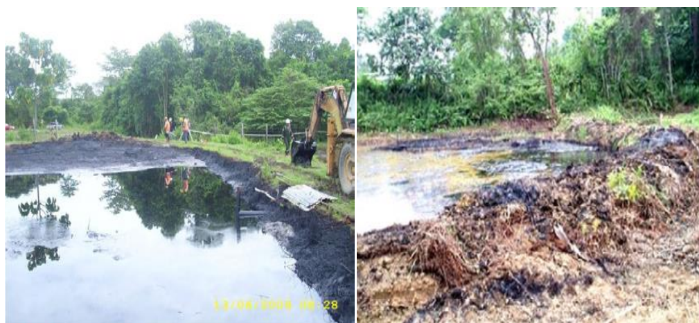
Figure 2.4: Untreated oily waste and oil sludge burial site (Edwan Kardena, 2015)
